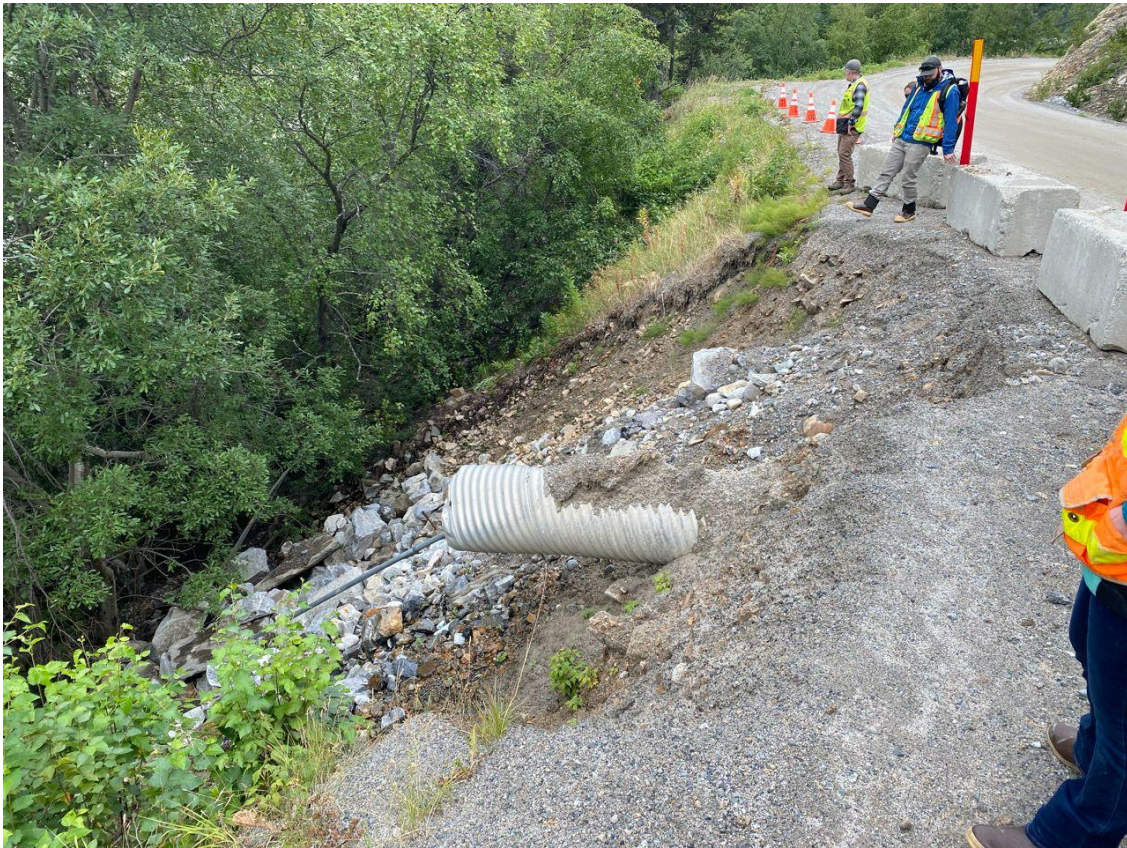
Slope erosion at Dyea Road MP 2.3.
